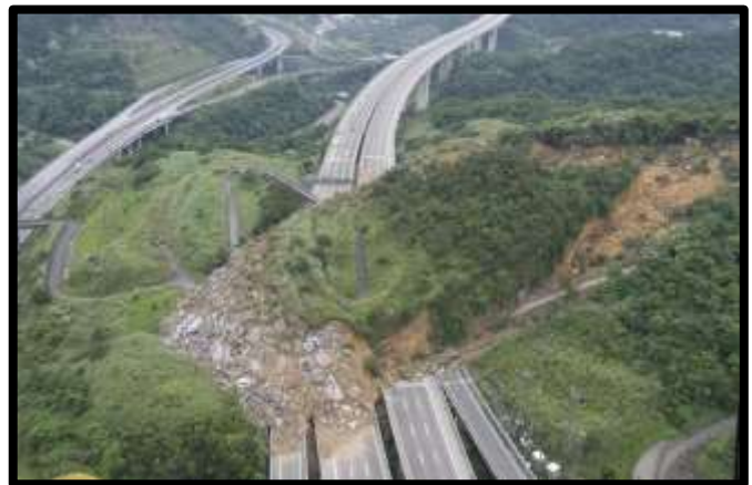
This is a landslide caused by a 6.5 earthquake in Taiwan.
